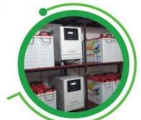
Water for battery inverter
